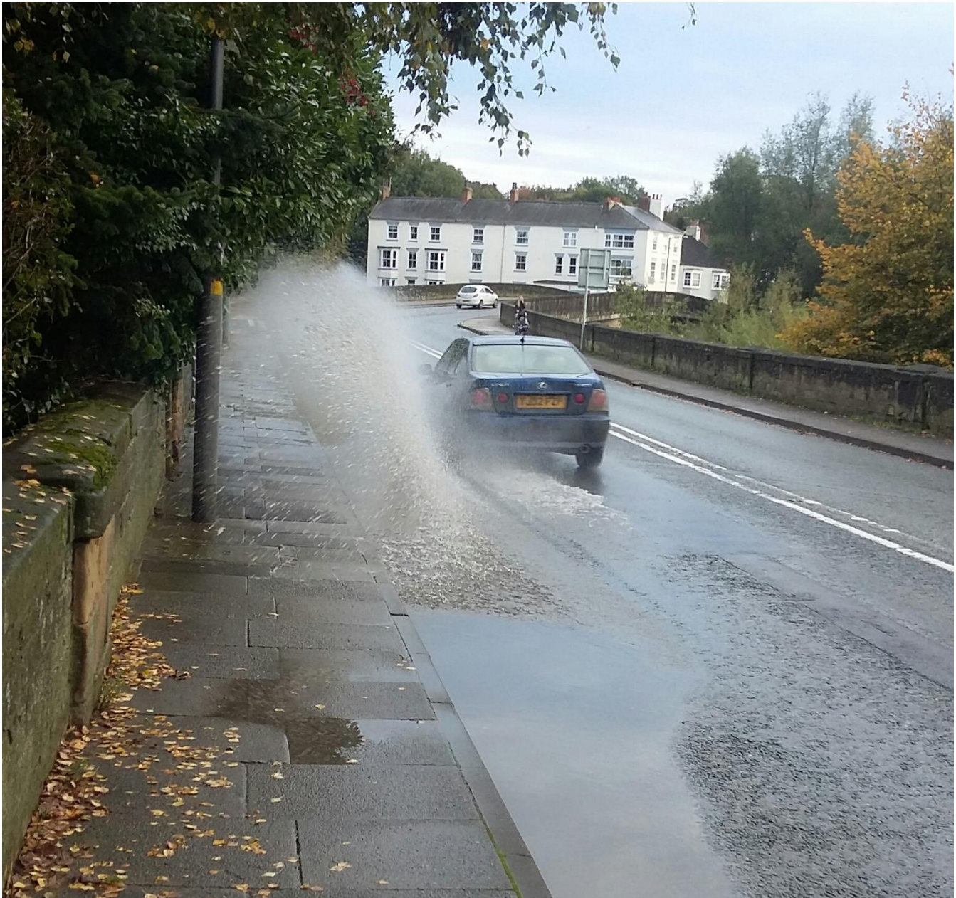
Surface-water flooding north of the bridge at 4.30 pm on Saturday (It was far worse an hour or two before; how many times has this problem been reported to NYCC?)
